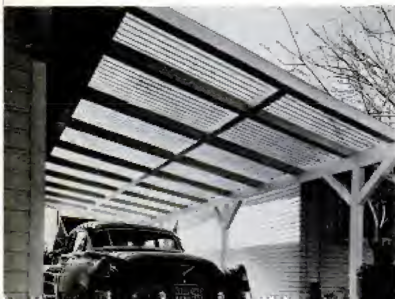
Absolutte Company of America photo Above, flat-type translucent plastic may be used in place of regular frosted glass where vision is not desired. Below, panels of corrugated plastic, 10 or 12 ft. long, simplify construction of a carport roof
